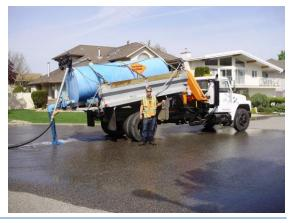
RWD has a flushing program that is primarily designed to remove mineralization build up. These minerals come out of suspension in the water during the disinfection process. The mineral residue tends to adhere to the pipe walls and only moves during higher flows from flushing or fire suppression.
